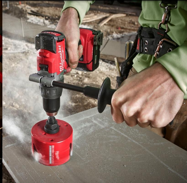
FIBER CEMENT SIDING
